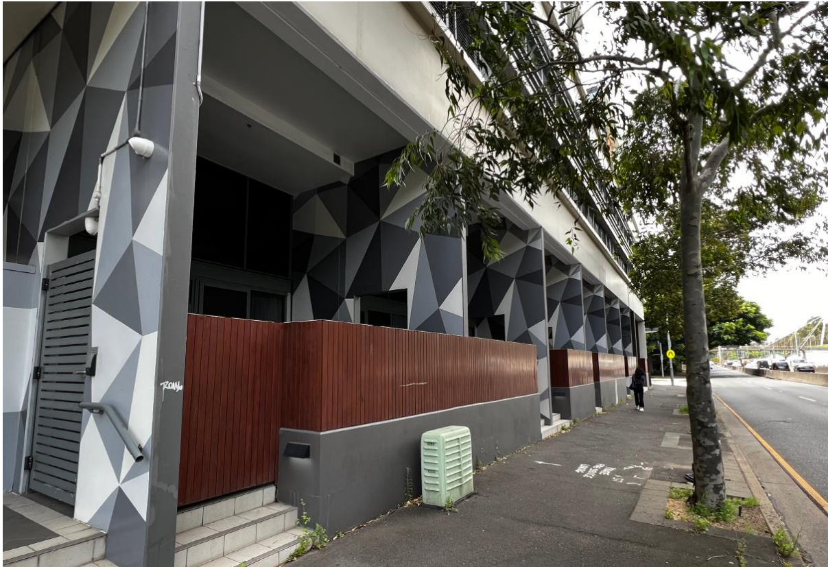
Figure 5: View of ground floor SOHO apartments fronting South Dowling Street
