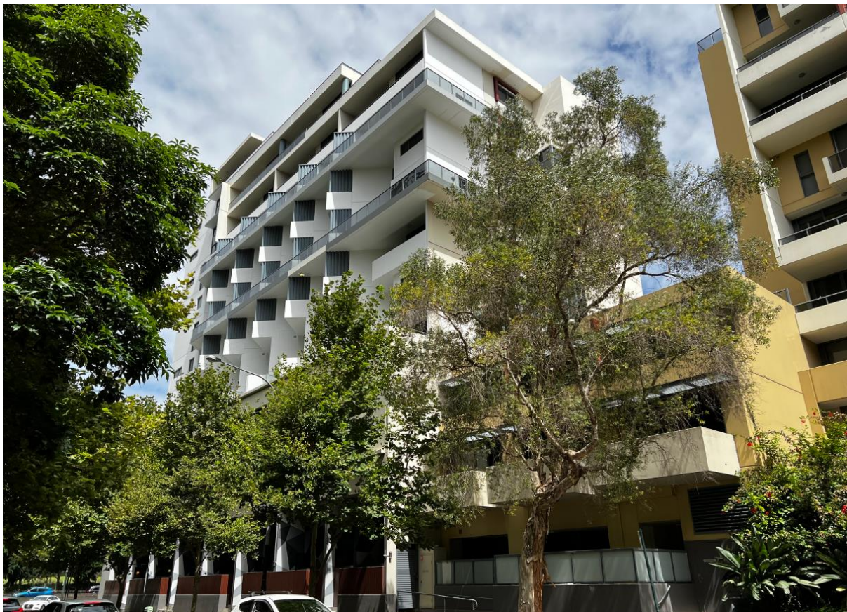
Figure 4: Site (Building C) viewed from Crescent Street
