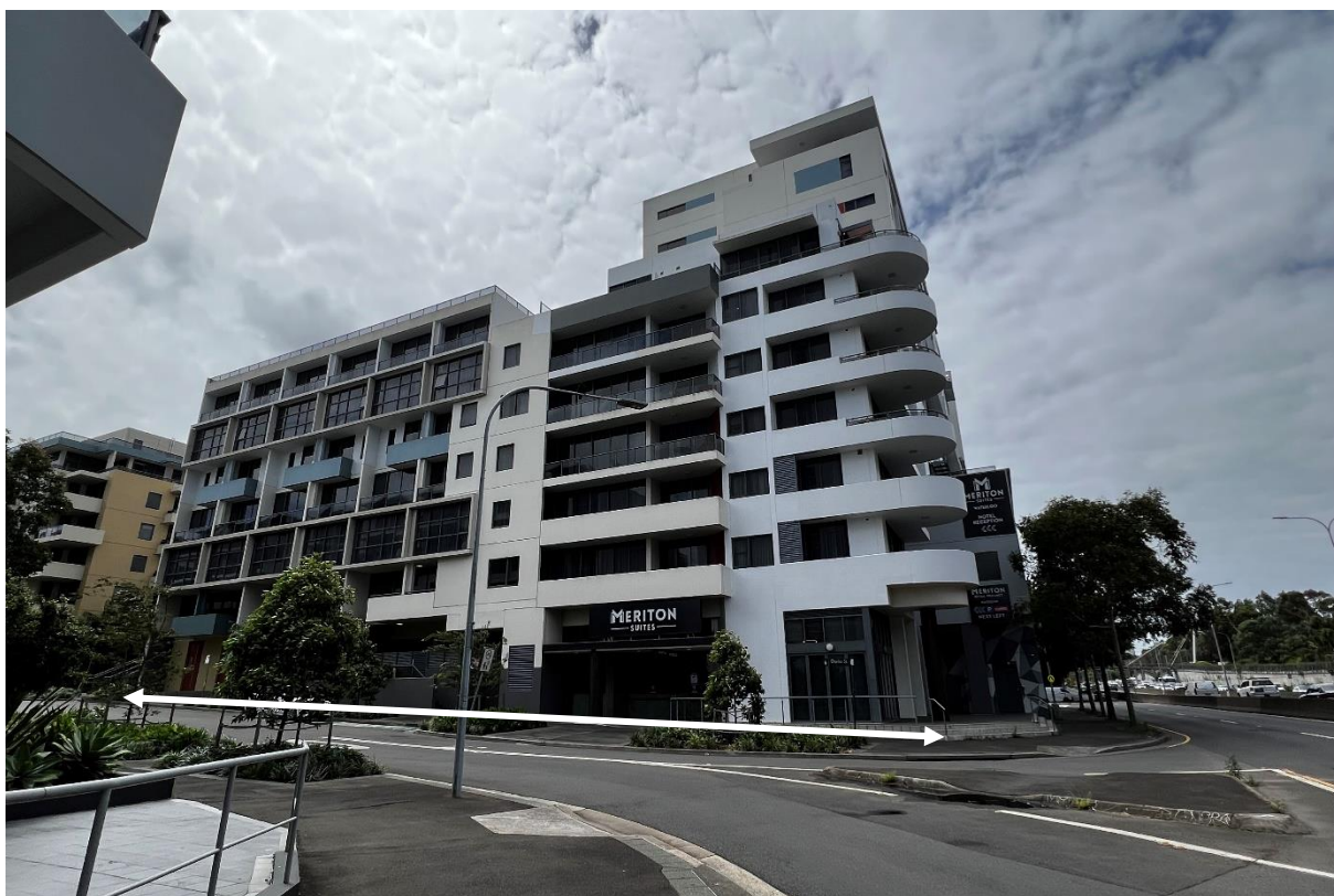
Figure 2: Site (Building D) viewed from the corner of Danks and South Dowling Streets
